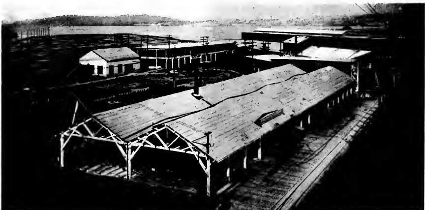
General view of the Ames plant showing the grouping of buildings and one corner of the building-ways.
